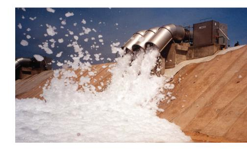
Expandol LT is a superior quality high expansion fire fighting foam concentrate for extinguishing and securing flammable hydrocarbon liquid fires.
